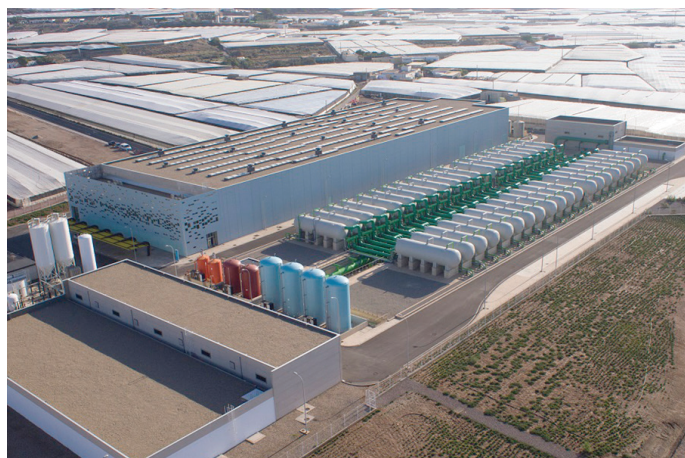
Figure 1: Campo de Dalías Desalination Facility
