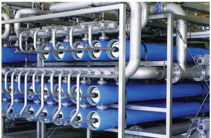
Figure 1: Low-pressure RO system at Löhnen drinking water plant
