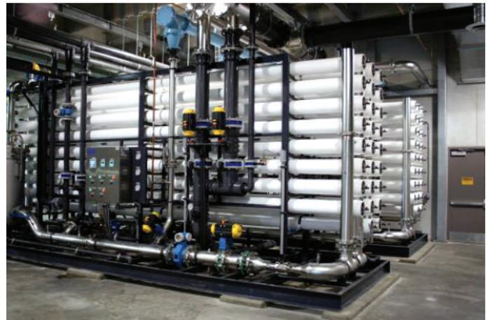
Figure 3 — RO skid using Toray RO membrane elements
