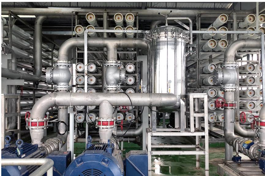
Figure 2 (left): Submerged PVDF UF skid
