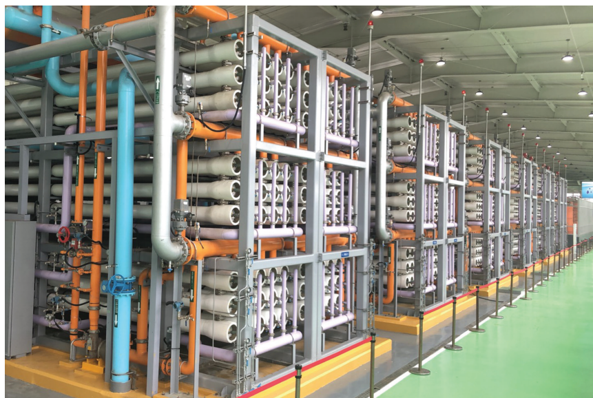
Figure 2: RO system containing Toray's low-fouling membrane elements
