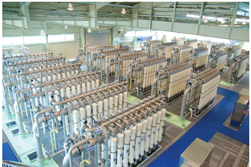
Figure 1: UF membrane system at Gongju WTP
