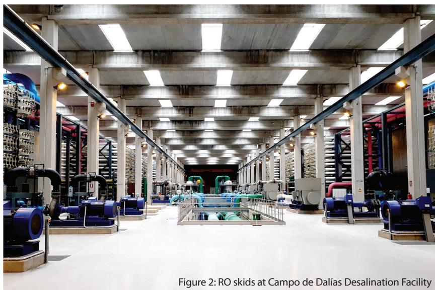
Figure 2: RO skids at Campo de Dalias Desalination Facility
