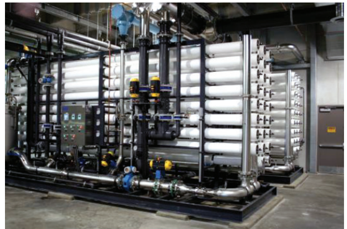
Figure 3 — RO skid using Toray's ROMEMBRA™ membrane elements
