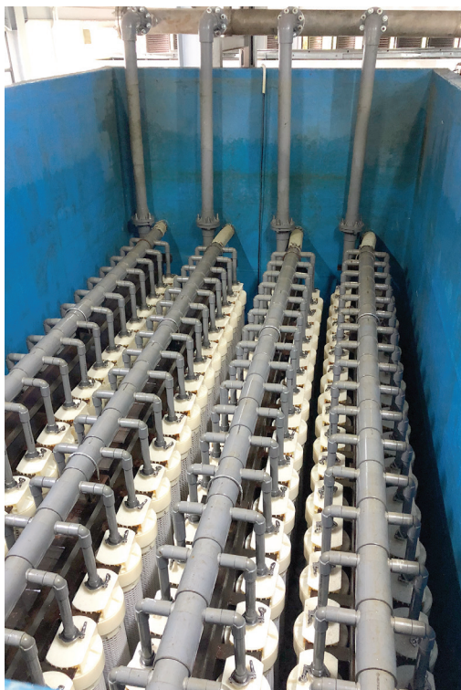
Figure 2 (left): Submerged PVDF UF skid Figure 3 (above): RO skids
