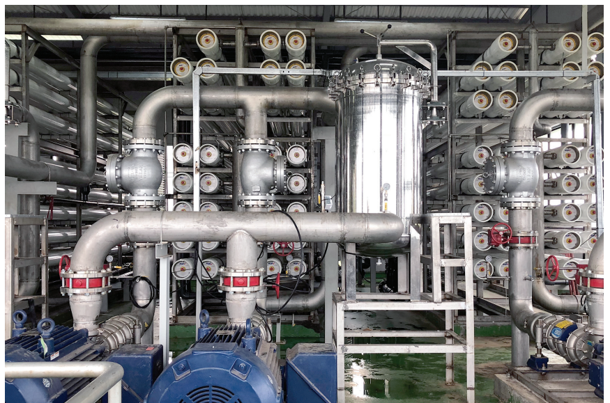
Figure 2 (left): Submerged PVDF UF skid Figure 3 (above): RO skids
