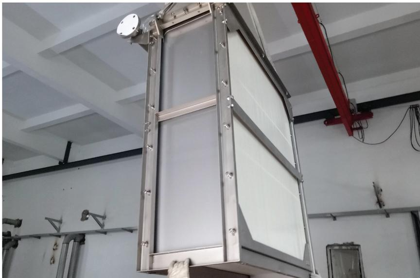
Figure 3: Installation of Toray MBR modules
