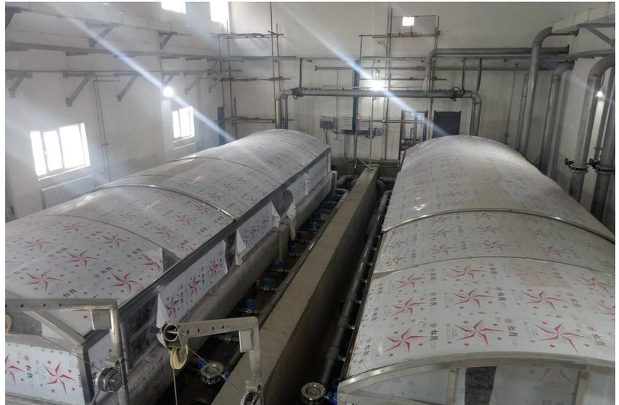
Figure 1: Tanks installed with Toray MBR modules at Lanzhou's bio-pharmaceutical facility
