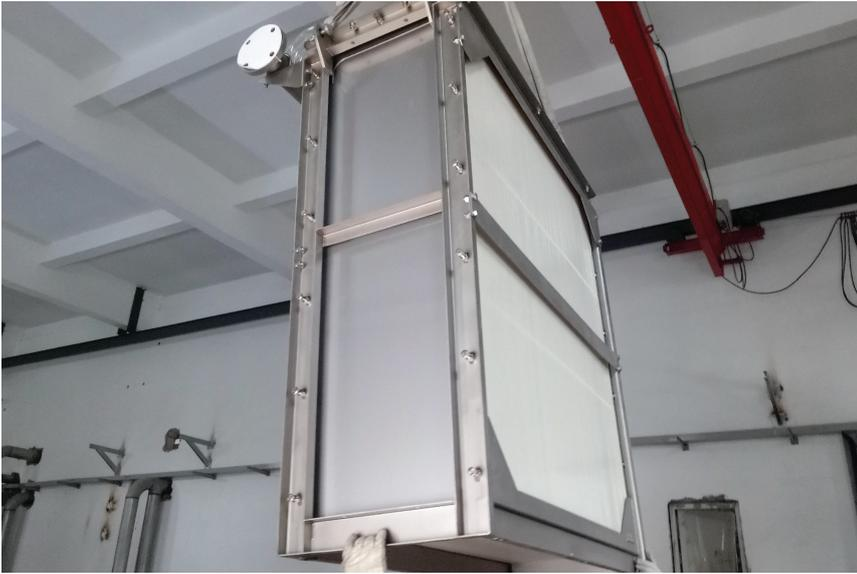
Figure 3: Installation of Toray MBR modules
