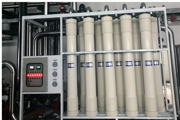
Figure 3: Toray UF system at Xiwu's thermal power plant
