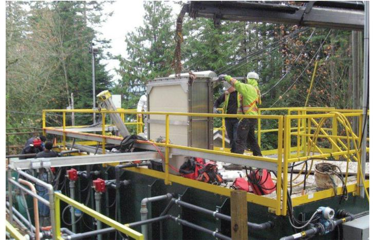
Figure 1: Installation of original Toray MBR
