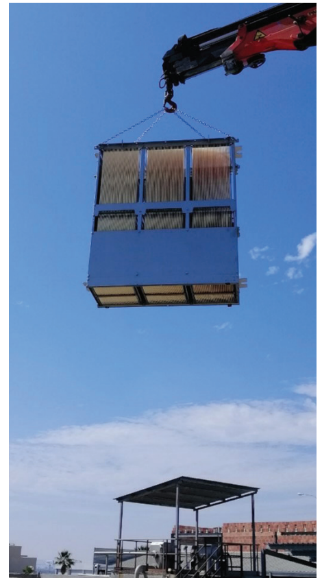
Figure 4: Installation of Toray MBR NHP Series
