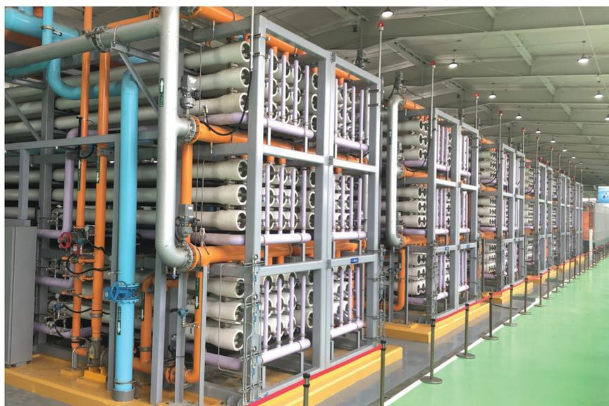
Figure 2: RO system containing Toray's low-fouling membrane elements
