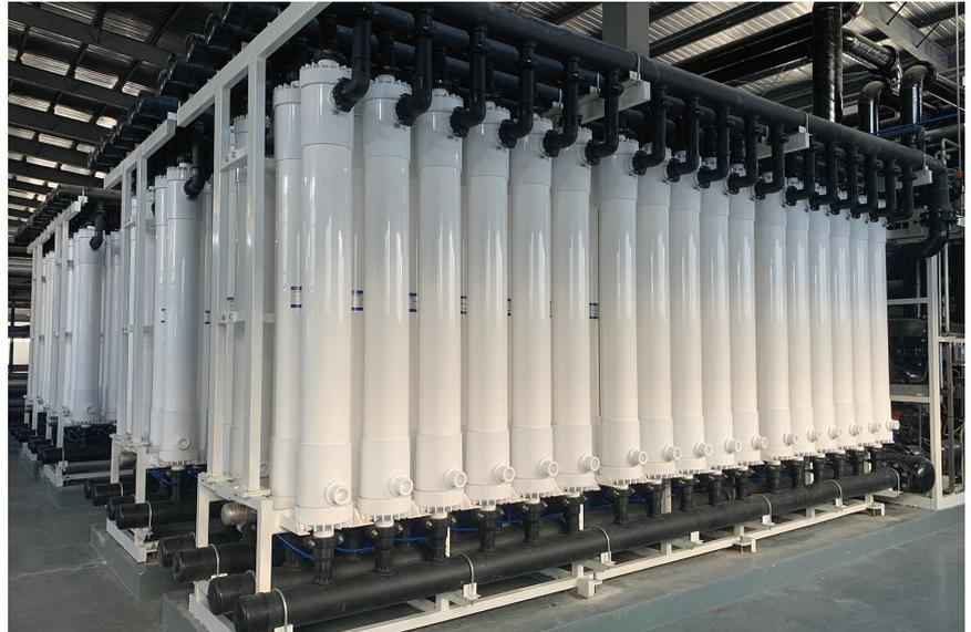
Figure 1: UF system at Wuxi installed with Toray HFUG-2020AN UF modules
