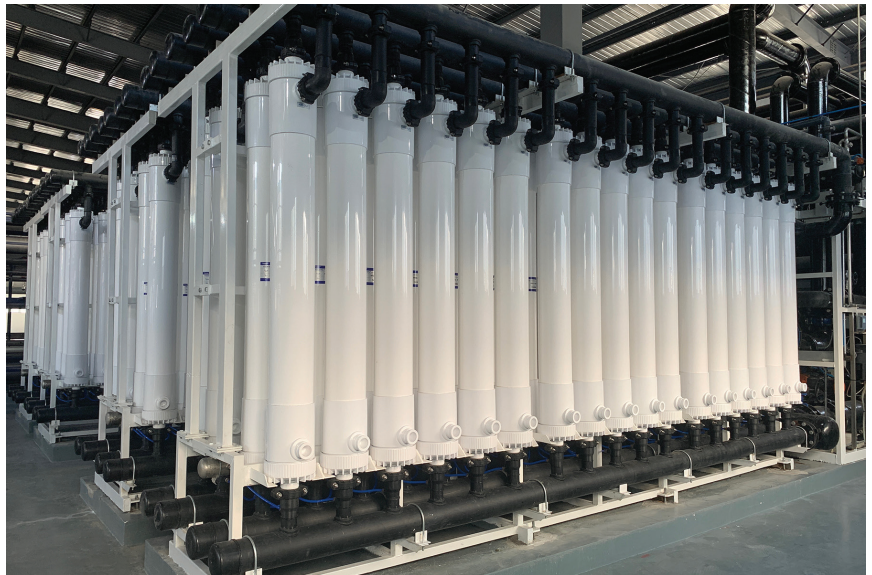
Figure 1: UF system at Wuxi installed with Toray HFUG-2020AN UF modules
