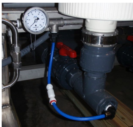
Poor location for air inject
