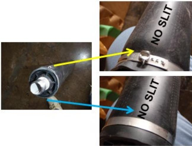
No Slit Area shall be located at top and bottom when connecting to the header pipe.
