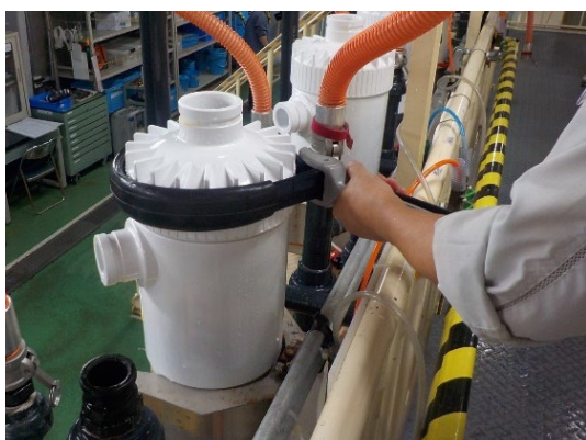
Figure 26: Opening Module Cap
