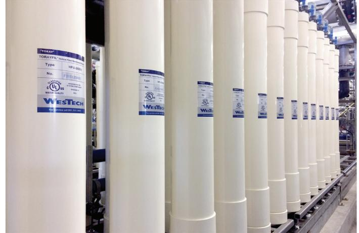
UF/RO system designed and constructed by WestTech Engineering ([WWW.WESTECH-INC.COM](http://WWW.WESTECH-INC.COM))
