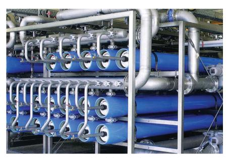
Figure 1: Low-pressure RO system at Löhnen drinking water plant
