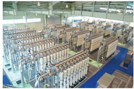
Figure 1: UF membrane system at Gongju WTP
