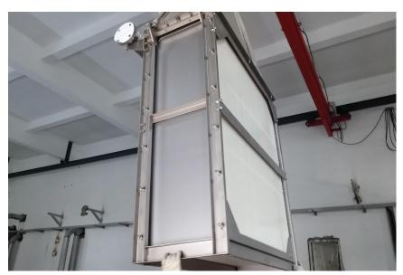
Figure 3: Installation of Toray MBR modules
