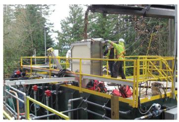
Figure 1: Installation of original Toray MBR
